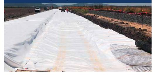
mastaTEX® Non-Woven is a non-woven needle-punched geotextile made from polyester, providing separation, filtration, protection or reinforcement functions in engineering projects. It enhances the performance and design life of granular layers by providing the filtration and separation functions.
